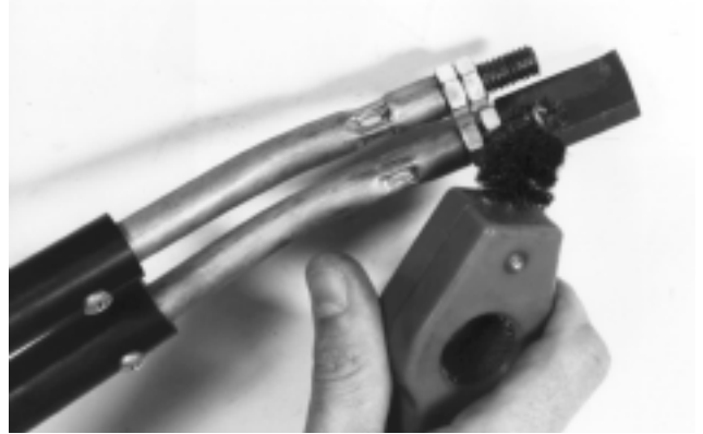
Figure 9 – Cleaning Threaded Stud
